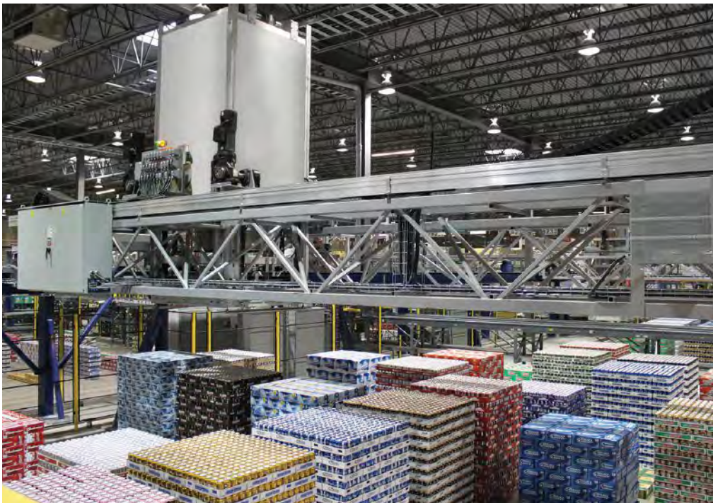
By analyzing real-time operational data, a systems integrator can often determine whether a system is operating as designed or if operating conditions have changed.
